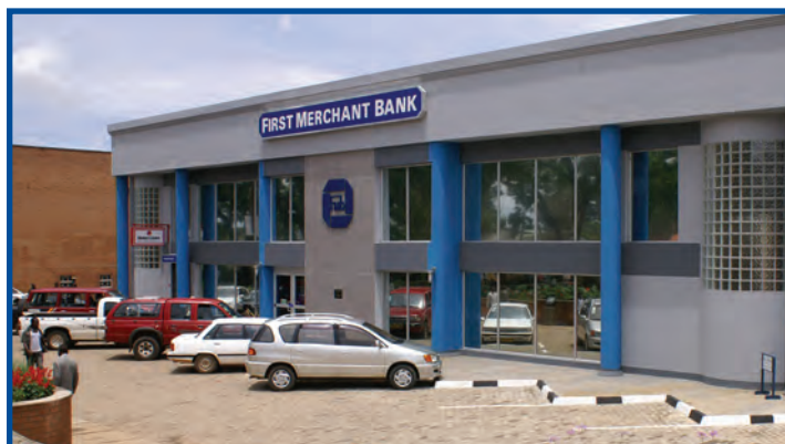
First Merchant Bank, Mzuzu Branch
